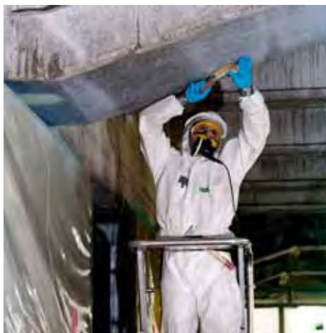
Figure 12: Asbestos removal 2
